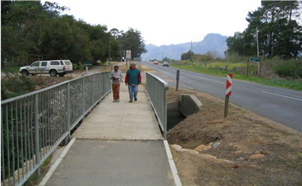
Figure 10: Example of a Separate NMT Bridge Structure next to the Roadway, NMT Guidelines (2015: 71)
